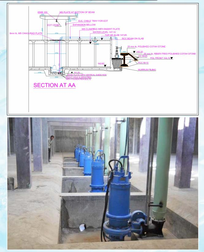
We are using "Aqua" make Submerged Centrifugal pumpsets (since 2011) for Clear as well Raw water applications. In our experience, as compared to HSCF or V7 pumps; Submerged CF pumps require
